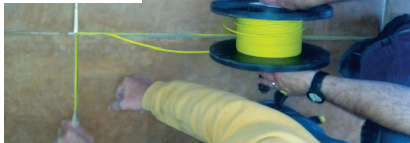
From top: The international symbol for the type of hearing loop installed at St. Mark's, Raleigh. At St. Mark's, the hearing loop wire is laid in the floor instead of in the walls as it is at many other locations. Photo courtesy of St. Mark's, Raleigh.
