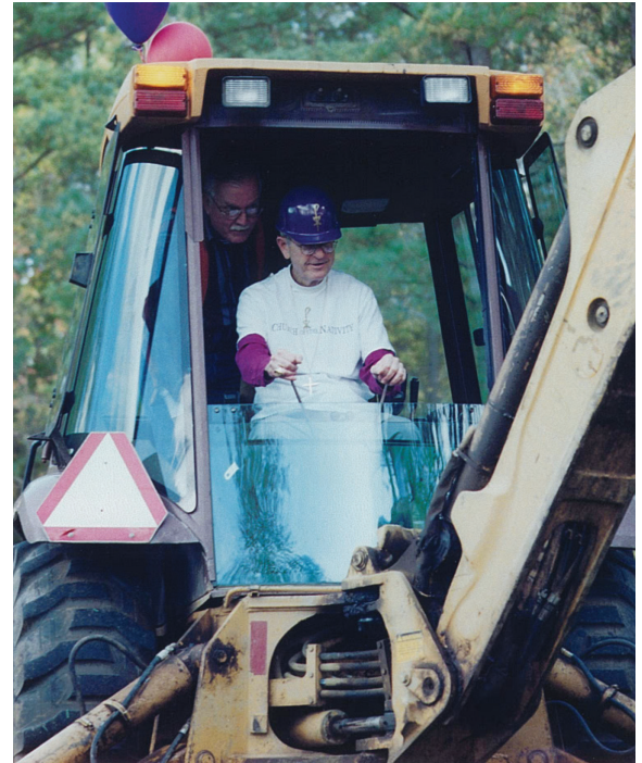
An archival photo of Bishop Robert Johnson operating a backhoe, breaking ground for a project at Nativity, Raleigh.
